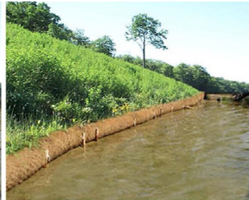
3 Months after the Coir log installation
